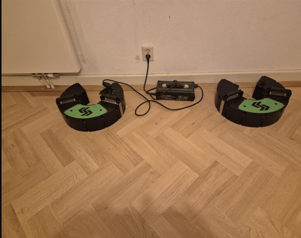
Kiwi Battery Packs with charger, on site
